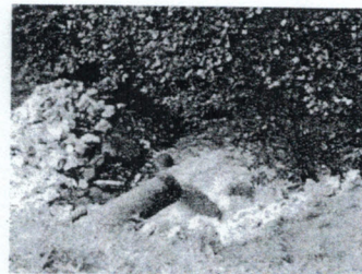
Rip-rap at Dixon Lake
